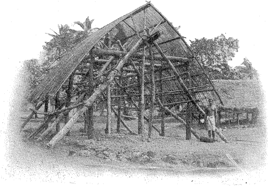
BEGINNING TO BUILD A SAMOAN HOUSE.
