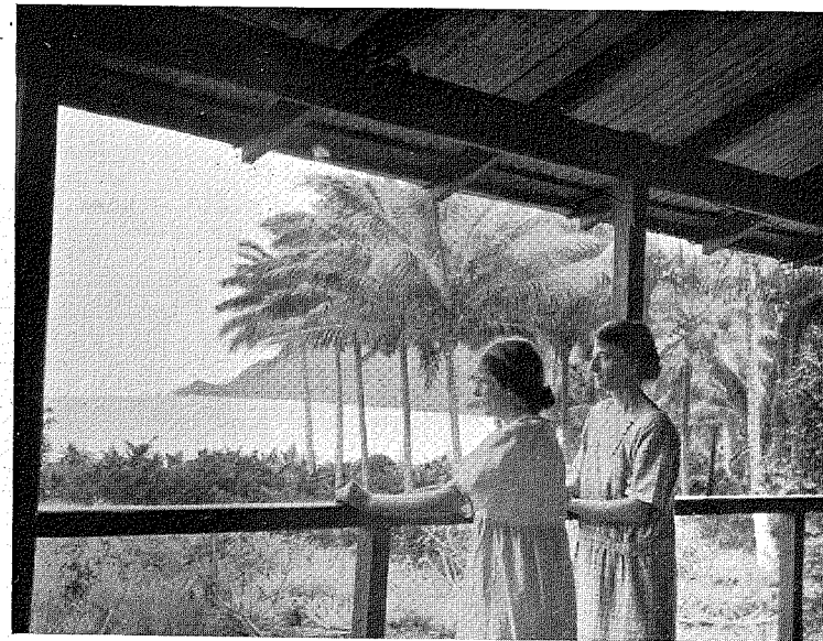
VIEW FROM VERANDAH.
